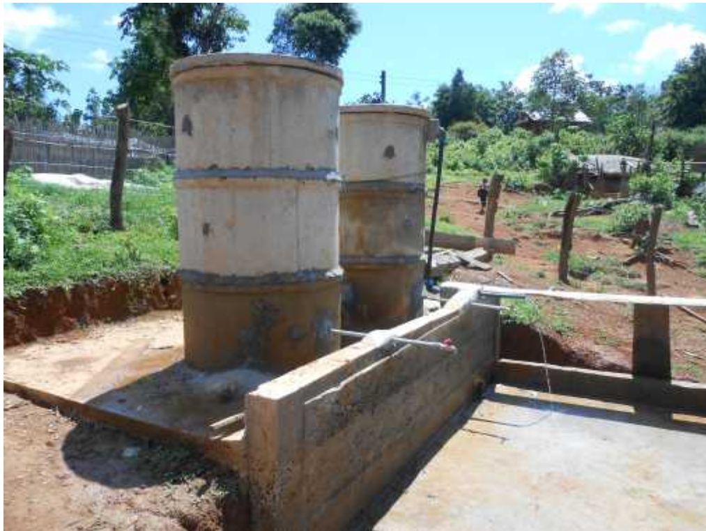
A nearly completed water point in the village.
