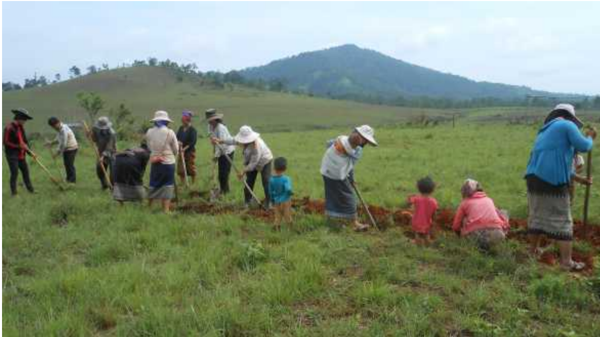
Mostly ladies starting to dig a 4 km long pipe trench. Note that the lady in the middle of the picture has her baby on her back. The men were away planting rice.
